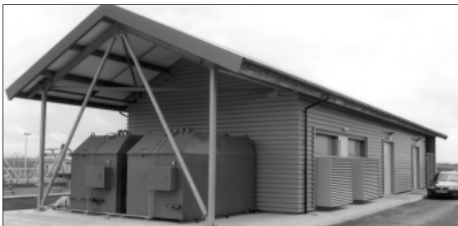
Good example of purpose made building to house two 1000 kVA generators with sound attenuators extending to the outside.
