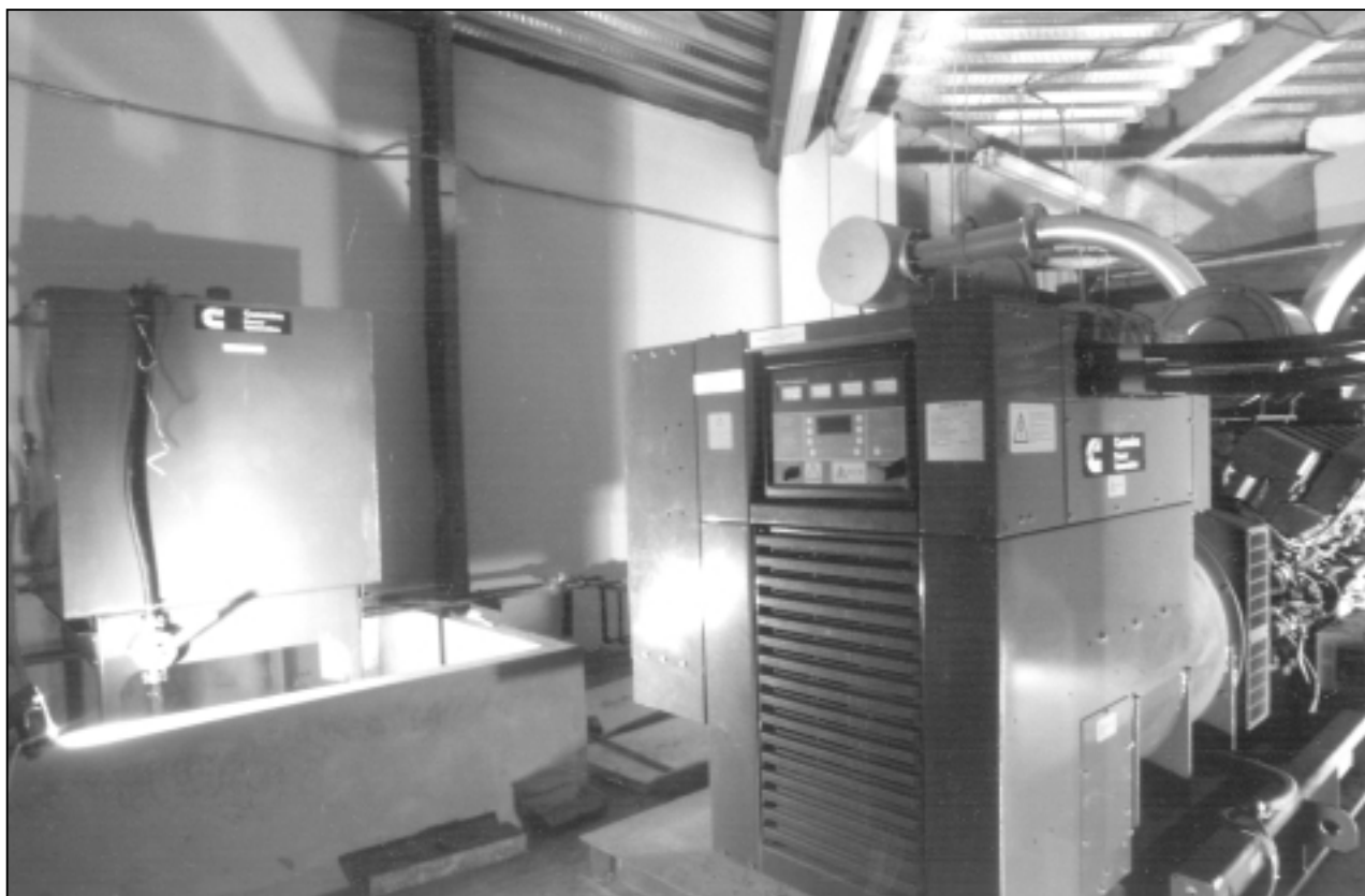
Example of a free standing 900 Litre fuel tank installed within a bund wall.
