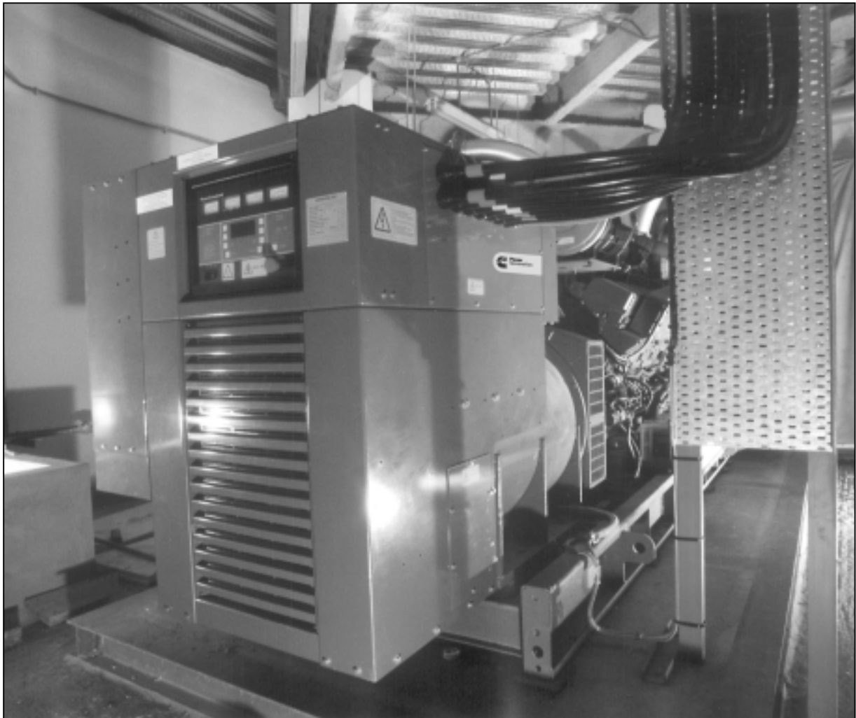
Flexible cable entry into control module and cable tray arrangement for side entry.
