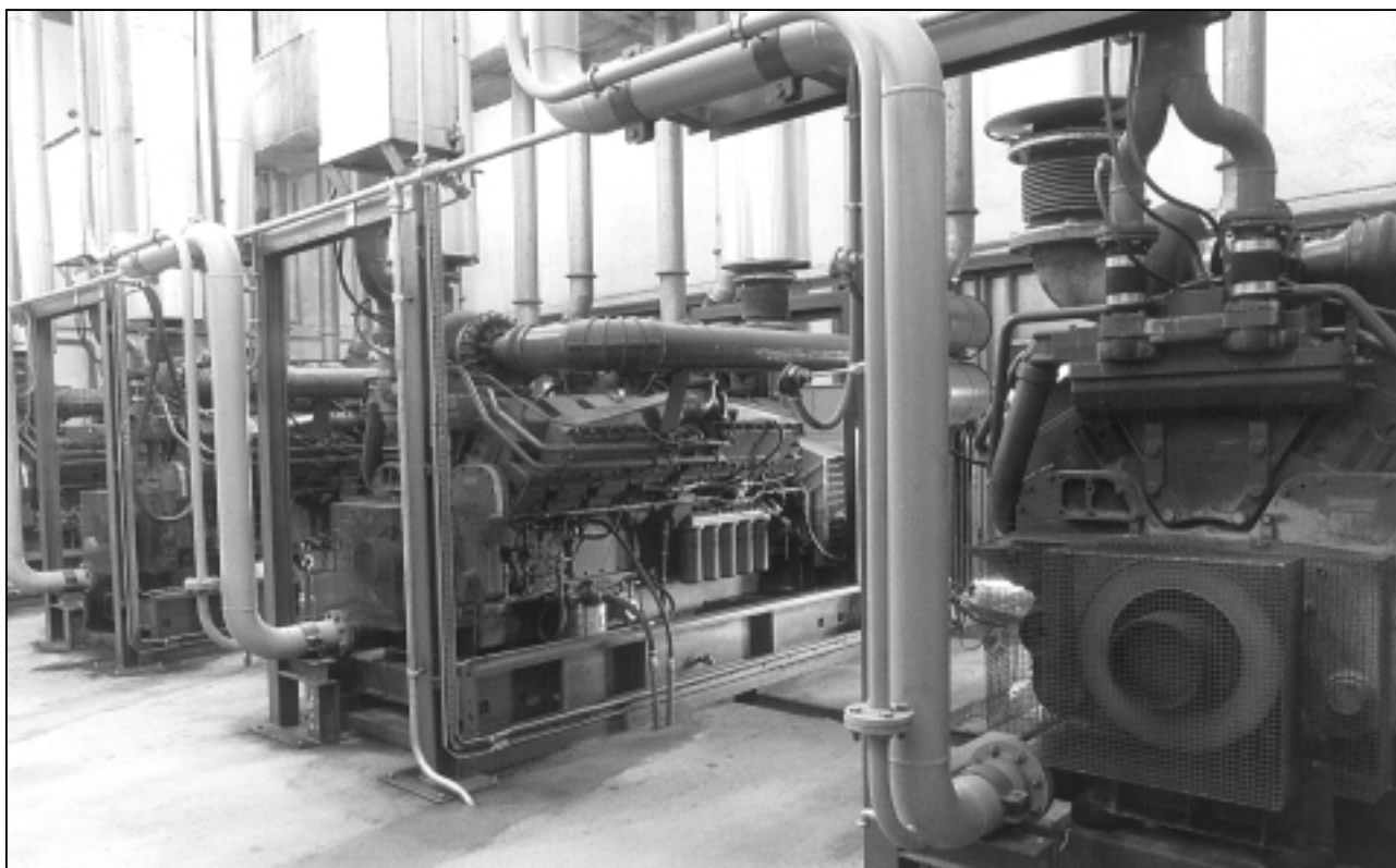
Four heat exchange cooled KTA50 Powered 1256 kVA sets run continuously for a factory in Spain.
