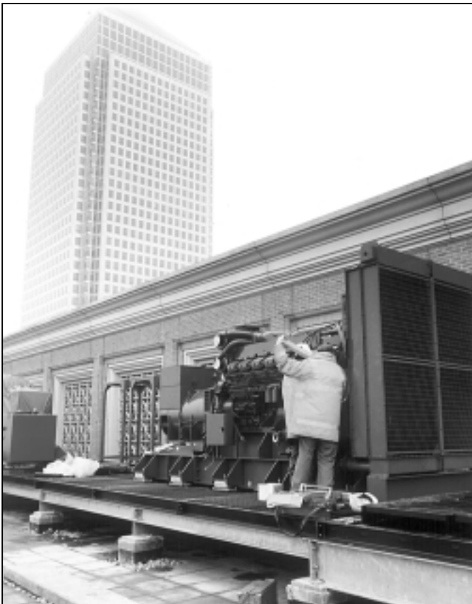
Unusual roof top (15 storeys high) installation for three 1500 kVA sets demands re-assembly of sets using rails and specially built A frame for transport and lifting.
