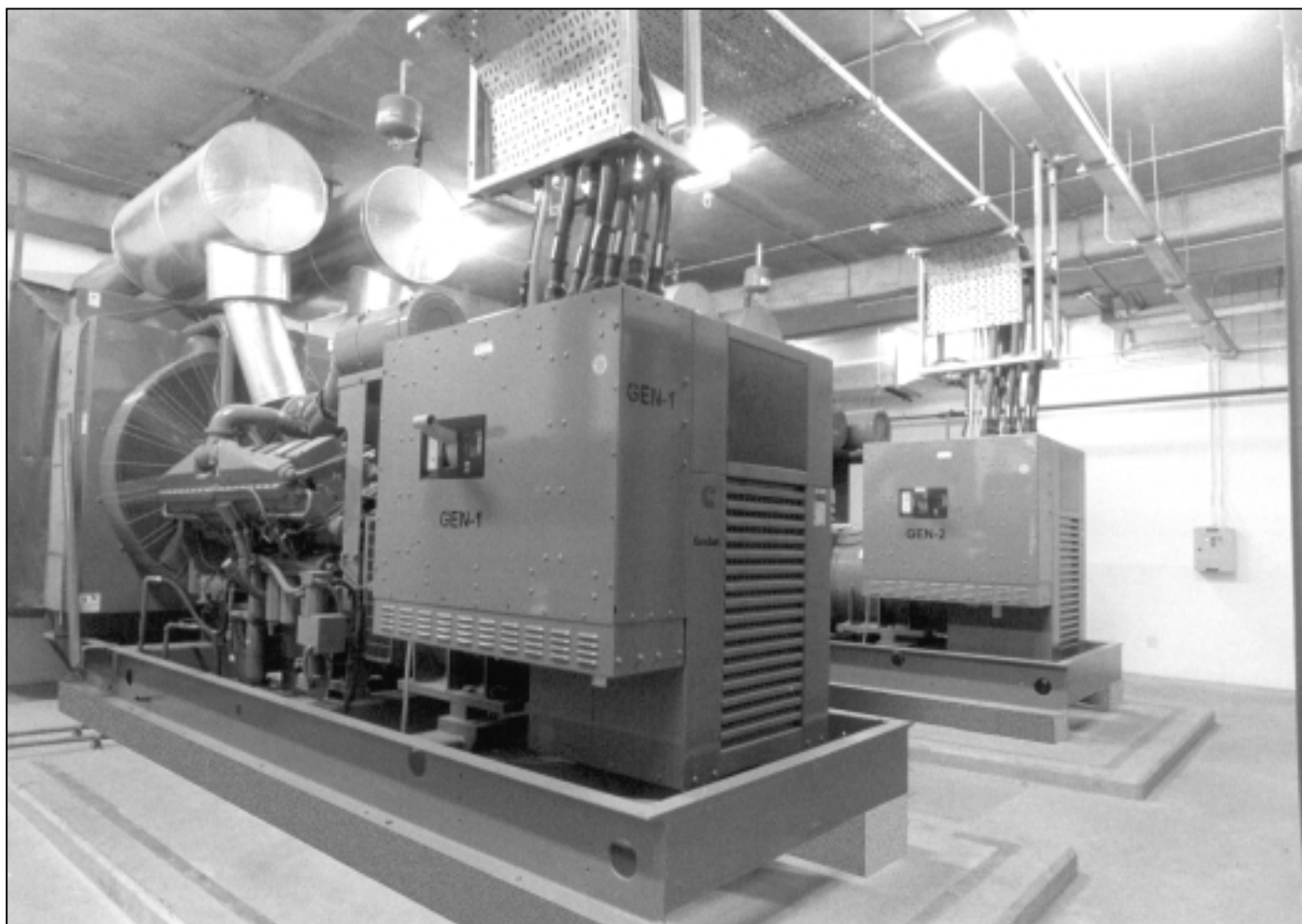
Top cable entry and overhead cable tray run between sets (1000 kVA sets).
