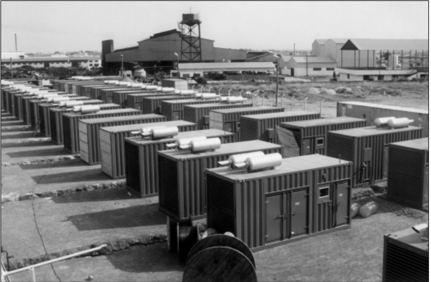
Typical 30 MW Cummins Power Station being installed on a site in Africa.
