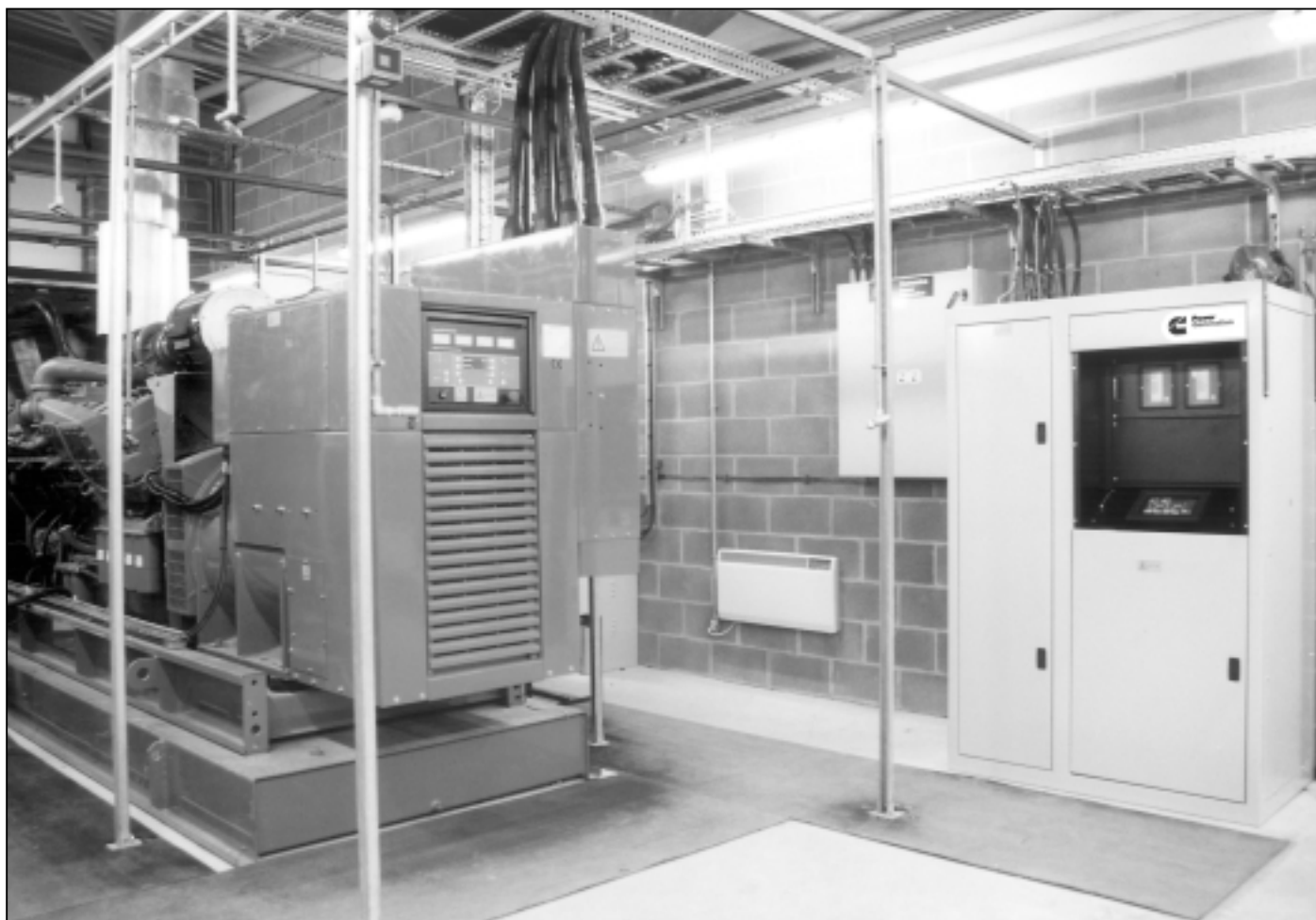
Cable installation into PCC module with Digital Master Control (DMC) cubicle and wall mounted changeover contactor box adjacent to set.
