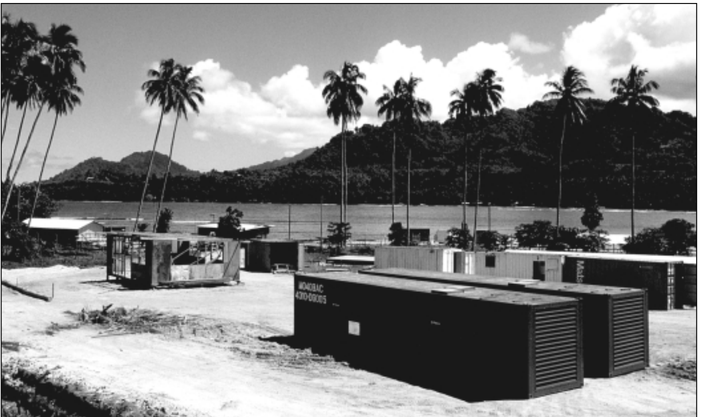
Large containerised generators for isolated locations provide a convenient package for transportation and fast installation.
