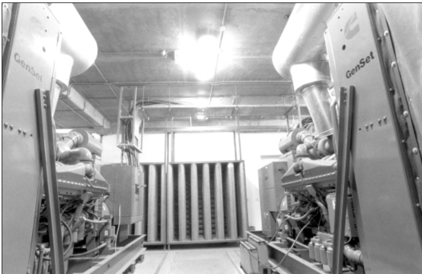
Sound attenuators inside a plant room for two 1256kVA CP1250-5 sets
