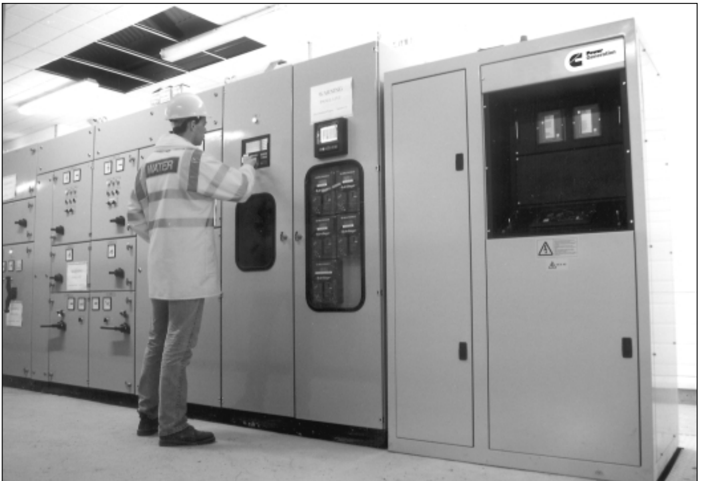
Digital Master Control Cubicle (DMC) installed with a water companies Switchboard Suite. Access to the DMC is all front entry.
