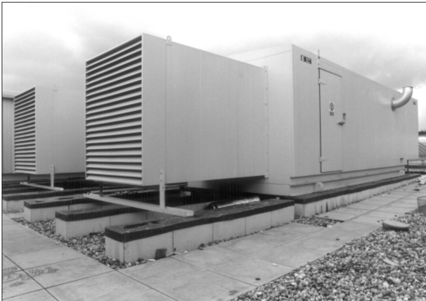
Two roof mounted super-silenced 1000 KVA sets with extended attenuators for a superstore provide a clean installation.
