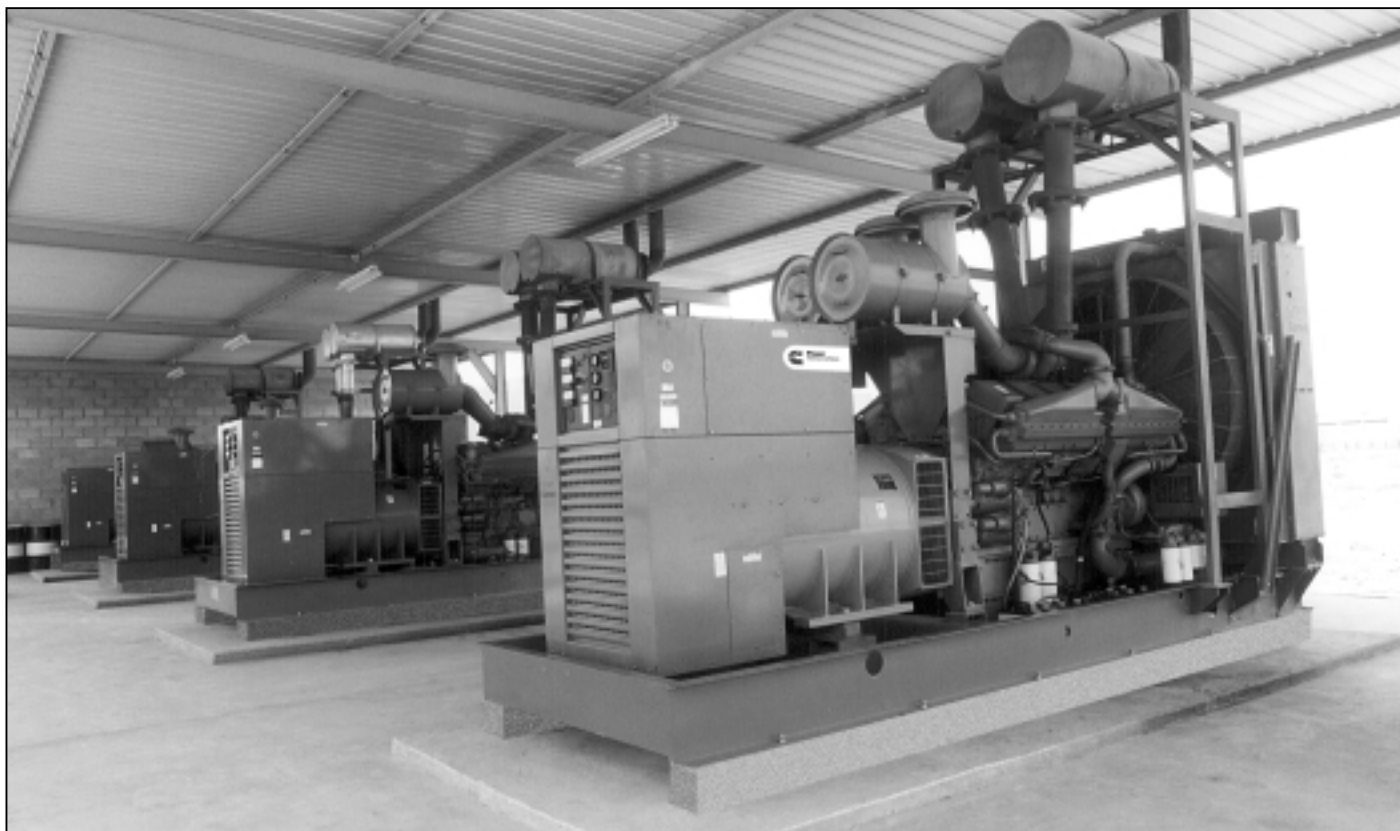
4 x 800 kVA Gen Sets in a ground level room installation with simple but effective exhaust run.
