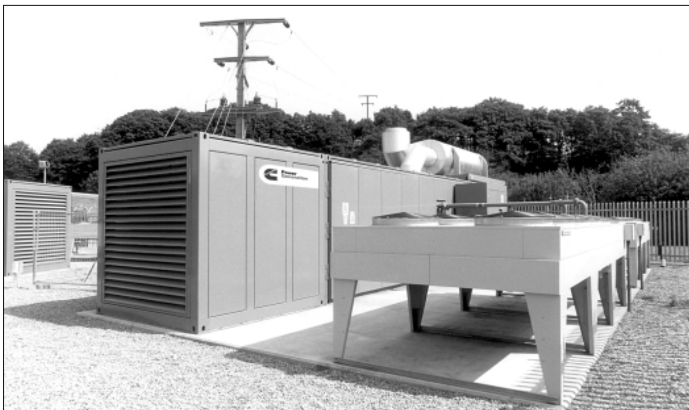
Fig. F7 Example of containerised style silenced enclosure for generators up to 2000 kVA
