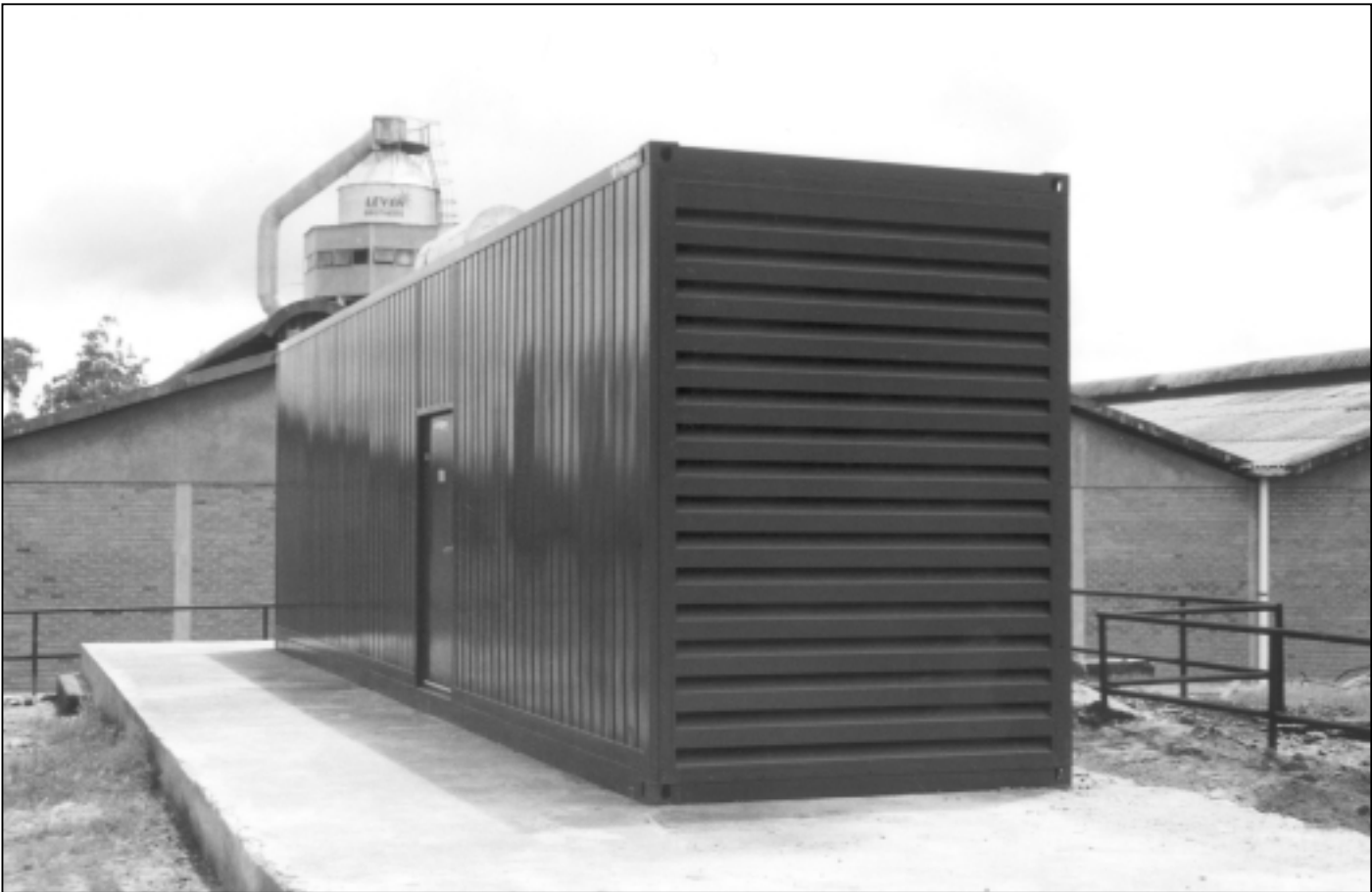
ISO container (9m) 30ft unit contains 600kVA emergency generator. Silenced to 75dB(A) at 1m
