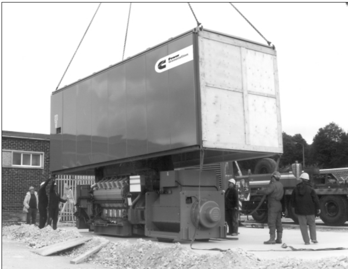
Drop over supersilenced enclosure for a 3700kVA Prime Power set sits on specially prepared concrete base
