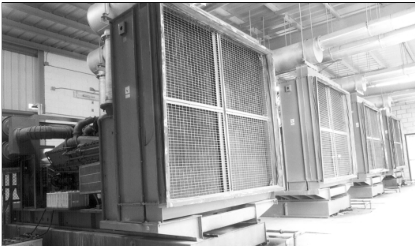
Four 1500 kVA sets with KTA50 engines running on base load operation in Saudi Arabia.
