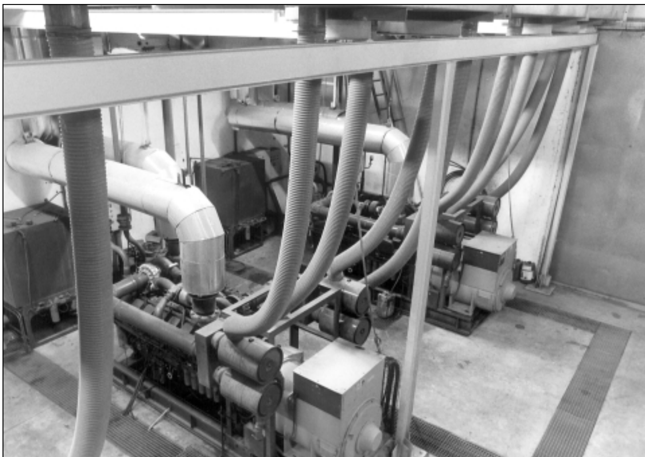
Where sets are in basement areas flexible trunking direct to the air intake cleaner ensures a cool supply.
