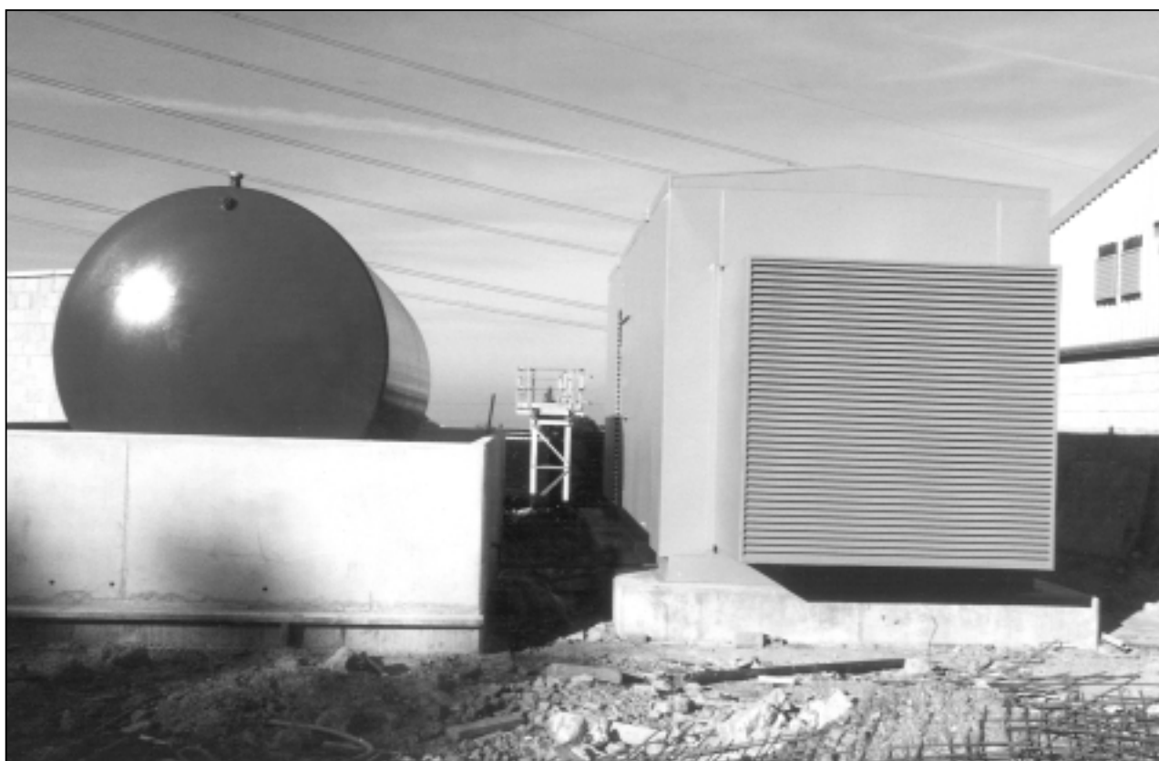
14000 Litre (3000 gallon) bulk fuel tank with a bund wall. Feeding a 500 kVA super silenced set with sufficient fuel for 6 days full load operation.
