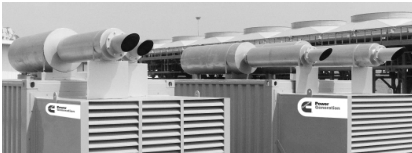
The combination of residential and a standard silencer as the tail pipe will effectively reduce exhaust noise.
