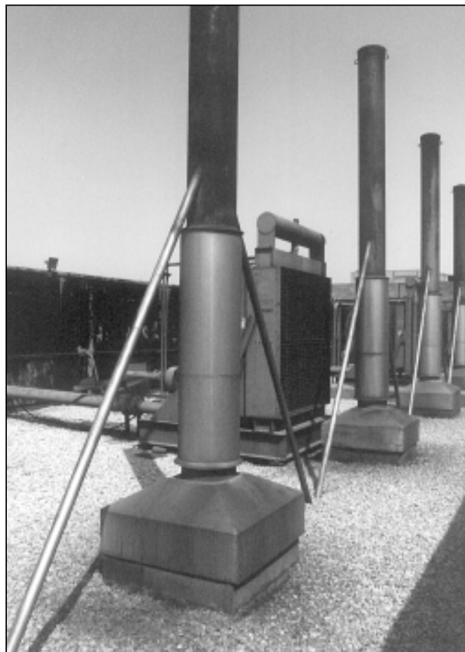
Roof mounted remote radiators for four 1000 kVA sets and extended exhaust tail pipes where space and air flow is restricted.
