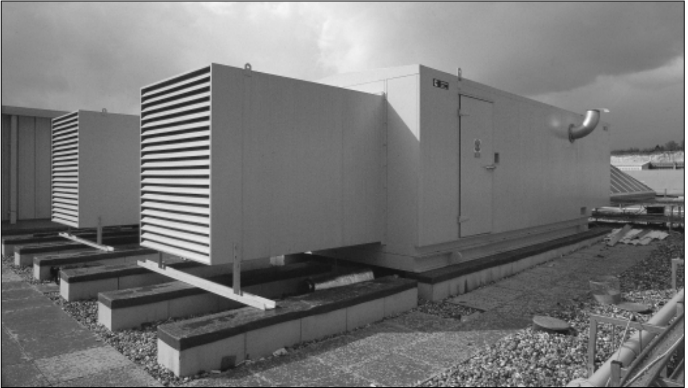
Two 1000kVA silenced standby sets with 'drop over' enclosures at roof top level eliminate many problems but create others
