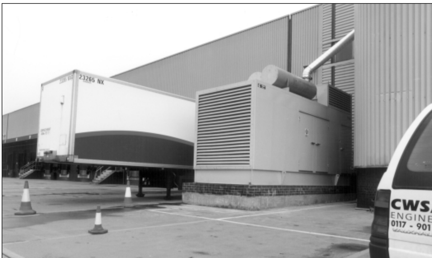
1000kVA Super Silenced (75dBA @ 1m) automatic standby set for major hypermarket chain warehouse
