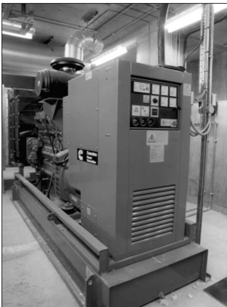
300 kVA standard generator with base fuel tank in typical plant room.
