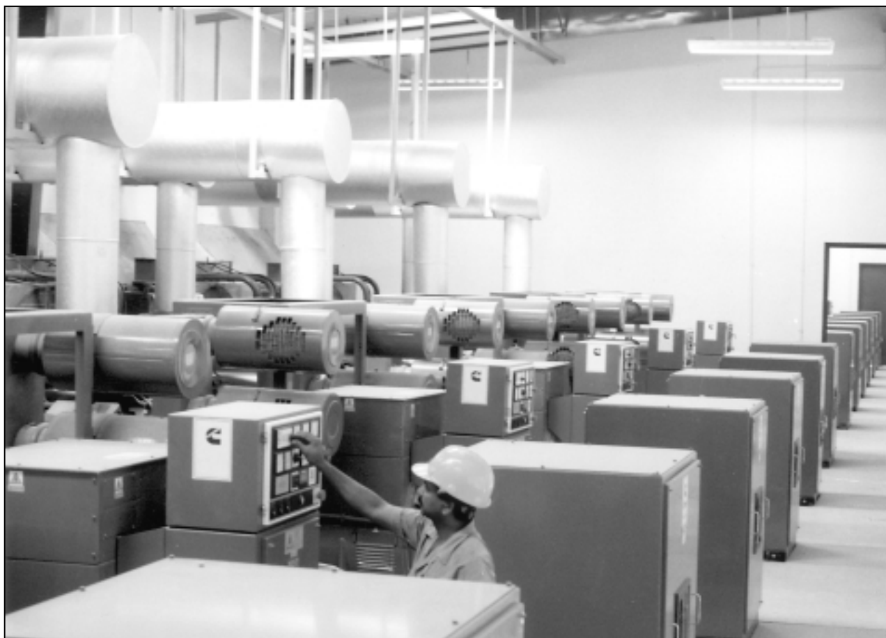
Twelve 1250 kVA sets working together as construction camp base power using the PCL control system.
