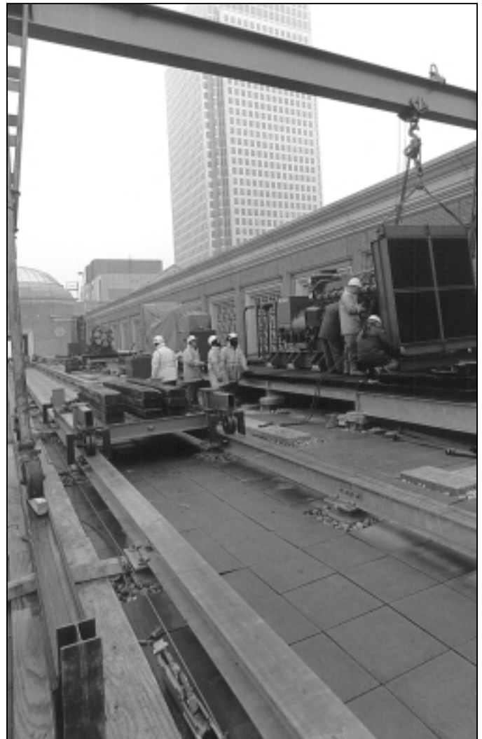
Unusual roof top (15 storeys high) installation for three 1500 kVA sets demands re-assembly of sets using rails and specially built A frame for transport and lifting.
