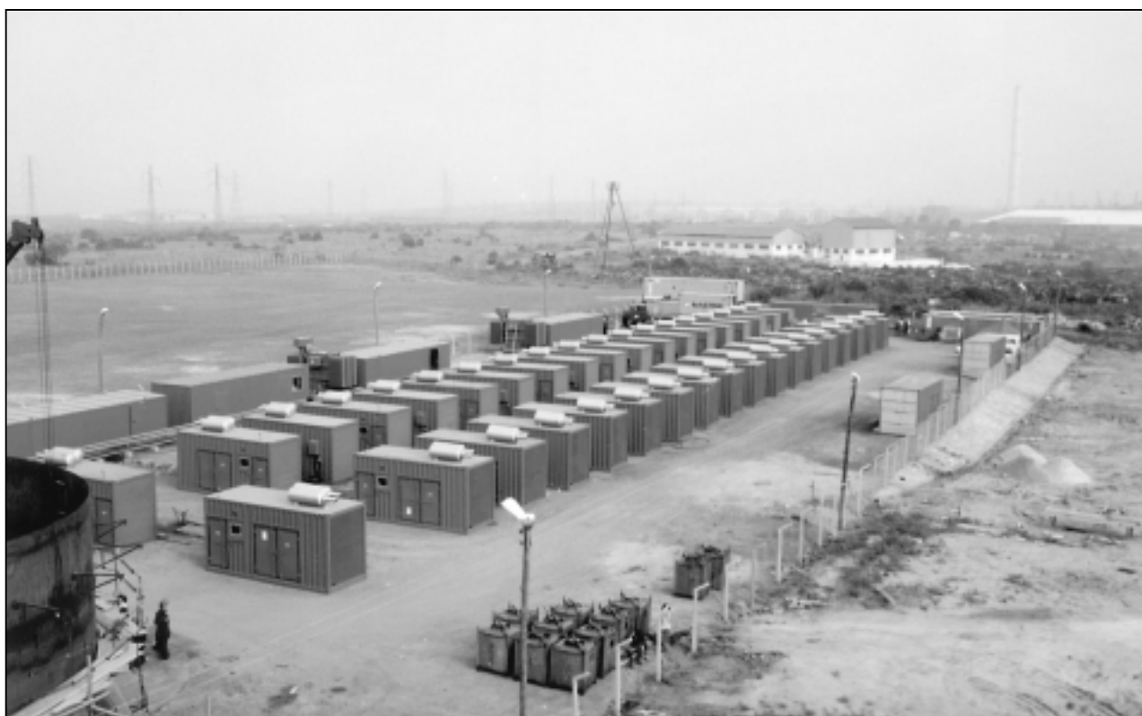
Thirty-nine 1125 kVA sets with KTA50 engines produce a combined 30MW of site power using PowerCommand Control (PCC) and Digital Master Control Systems when all operating in parallel.
