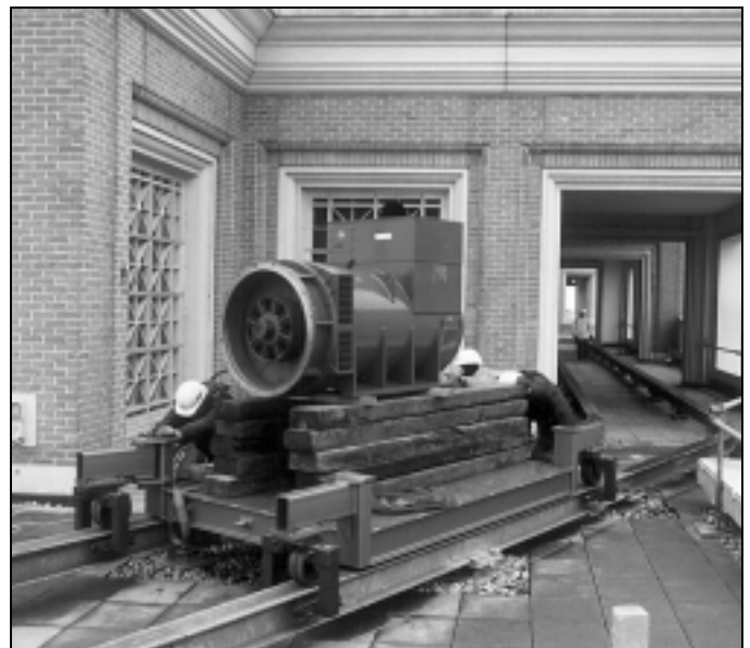
Unusual roof top (15 storeys high) installation for three 1500 kVA sets demands re-assembly of sets using rails and specially built A frame for transport and lifting.
